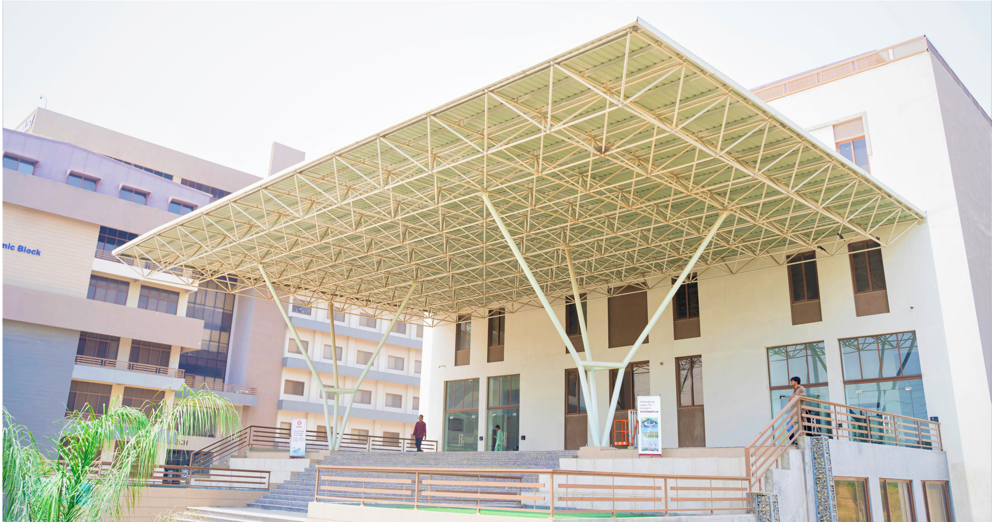
Structure Type: Space Frame Structure
